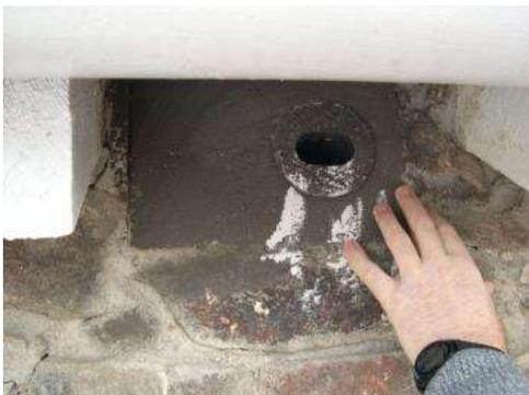
Plastic soffits and gutters have been fitted to this re-roofed house. Holes have been cut in the soffits close to the wall to provide access for the Swifts to their nests in the eaves.
